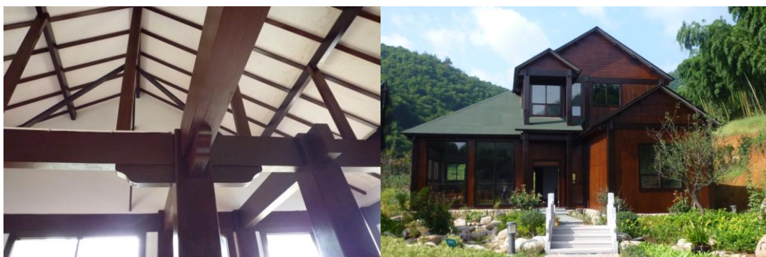
SWB as Structural Building Material in the Bamboo House, Anji County, China
